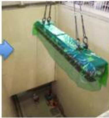
move into tunnel
