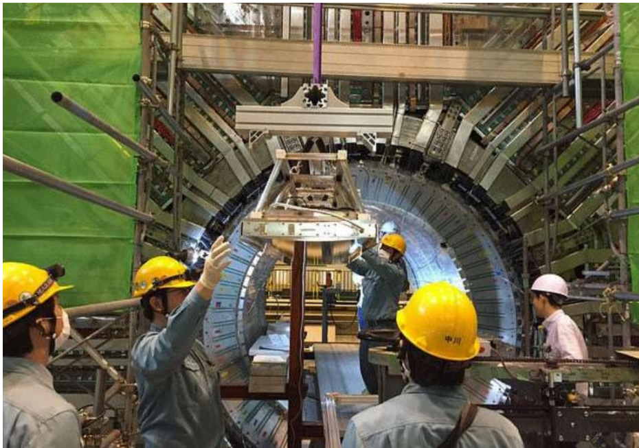
Figure 2.24.: Installation of the first iTOP module in Belle II
